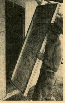
ied at "C" on Fig. 6.) Be sure to put glue and blanket stripping at all joints. All roof panels are put on except the last one. This panel is left off until the main door is cut out.
